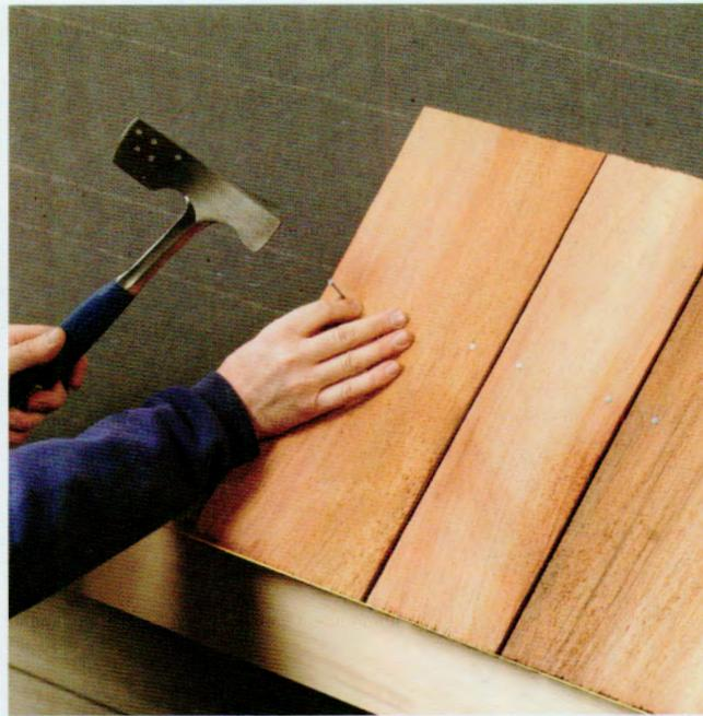
**2** Install a starter shake so it overhangs the eaves and rake edge by 1 1/2". Do the same on the opposite side of the roof. Run a taut string between the bottom edges of the two shakes. Install the remaining shakes in the starter row, aligning the bottoms with the string. Keep the manufacturer's recommended distance between shakes, usually 3/8" to 5/8".
