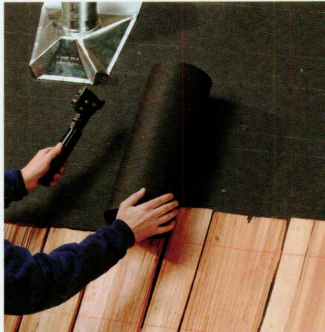
**4** Snap a chalk line over the first course of shakes at the exposure line. Snap a second line at a distance that's twice the exposure rate. Staple an 18"-wide strip of felt paper at the second line. Overlap felt paper vertical seams by 4". Install the second course of shakes at the exposure line, offsetting joints by 1 1/2" minimum. Install remaining courses the same way.
