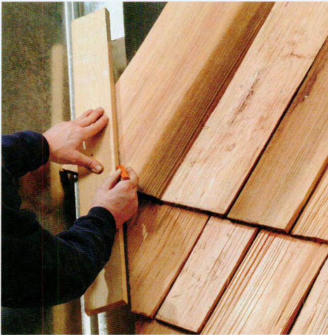
**5** Set shakes in place along valleys, but don't nail them. Hold a 1 × 4 against the center of the valley flashing without nailing it. Place it over the shakes to use as a guide for marking the angle of the valley. Cut the shakes, using a circular saw, then install.
