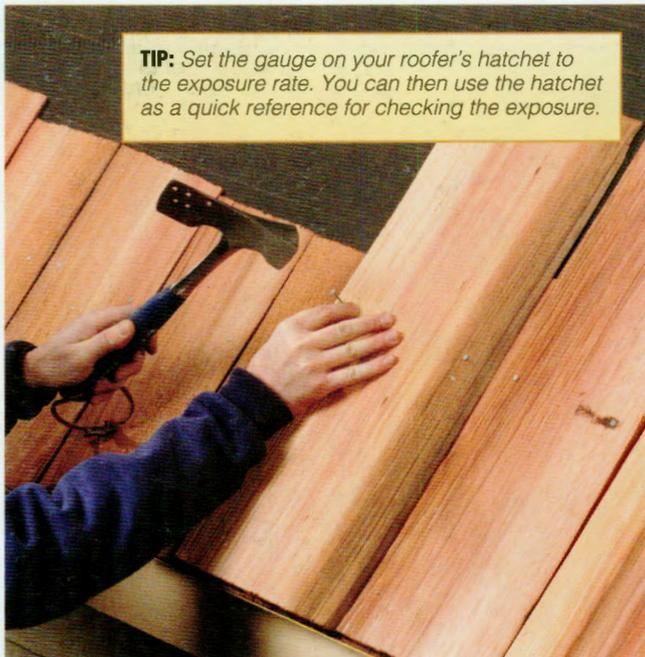
**3** Set the first course of shakes over the starter row, aligning the shakes along the rake ends and bottoms. Joints between shakes must overlap by at least 1 1/2". Drive two nails in each shake, 3/4" to 1" from the edges, and 1 1/2" to 2" above the exposure line. Use the hatchet to rip shakes to fit.
