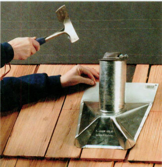
**7** Notch shakes to fit around a plumbing stack, using a jig saw, then install a course of shakes below the stack. Apply roofing cement to the underside of the stack flashing, then place it over the stack and over the shakes. Nail the flashing along the edges.
