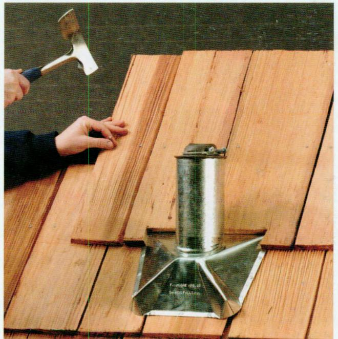
**8** Overlap the exposed flashing with the next row of shakes. Cut notches in the shakes to fit around the stack, keeping a 1" gap between the stack and shakes.
