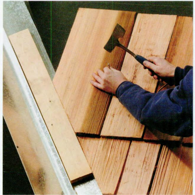
**6** Use the 1 × 4 to align the edge of the shakes along the valley. Keep the 1 × 4 butted against the valley center, and place the edge of the shake along the edge of the board. Avoid nailing through the valley flashing when installing the shakes.
