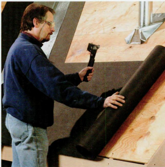
**1** Prepare the roof decking by installing valley flashing at all valleys (pages 66 to 67). Apply felt paper underlayment to the first 36" of the roof deck. Note: Depending on your climate and building codes, you may want to install ice and water shield for this step rather than felt paper.
