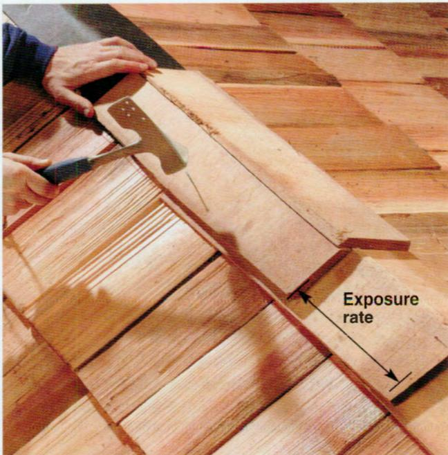
**15** Set a ridge cap along the chalk line, flush with the edge of the roof, to serve as the starter. Install with two nails. Place a cap directly on top of the starter cap, and nail in place. Install caps along the remainder of the ridge, alternating the overlap pattern. The exposure rate should be the same as the roof shakes. Nails should penetrate the roof decking by  $\frac{1}{2}$ ".
